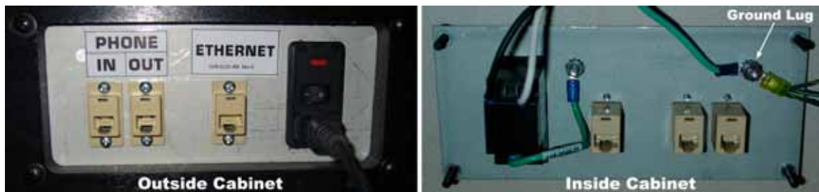
Figure 39. AC Power Plate
